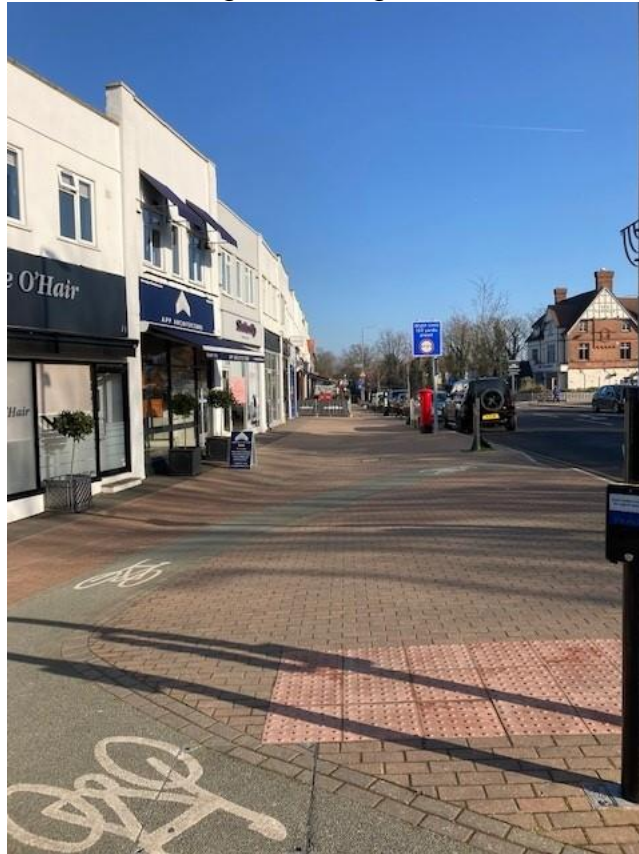
Photo 3: application site looking northeast along Red Lodge Road
